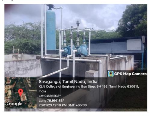
This plant is located nearer to the Ladies Hostel. Here drainage water is filtered and recycled by various treatments. This recycled water is used for watering the plants in gardens.
