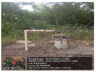
This bore well is located into an underground in the various places of our campus such as Backside of Automobile block, Nearer to Indoor Stadium, At Gents hostel, Nearer to College main gate etc . The 5HP electrical pumps are used in our campus to pump out the water from the bore wells.
